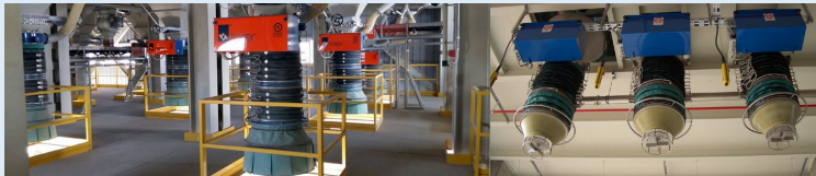
Figure 2 – Loading Bellows, which form part of an extensive product range SAVECO provides for Industrial & Municipal WWT sectors.
